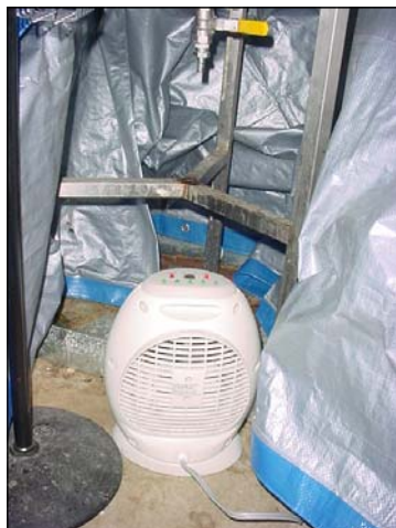
Here's the heater inside the tarp. Be on the safe side and make sure the tarp doesn't touch the heater.
